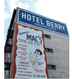
Jamboree Housing Corp., began renovation of the Hotel Berry earlier this year.
